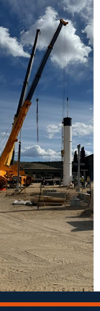
To overcome the challenges of Colorado's cold climate and ensure timely project execution, Audubon established strict safety protocols, sourced specialized equipment and materials, prewarmed components, and prepared indoor storage facilities, alongside scheduling construction around weather impact. We also provided crucial construction support with foundational helical piles, heat tracing, and insulation for piping, ensuring long-term protection of our client's assets.
