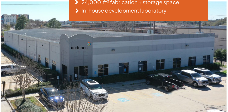
Audubon Manufacturing and Technology Center, Houston, Texas
